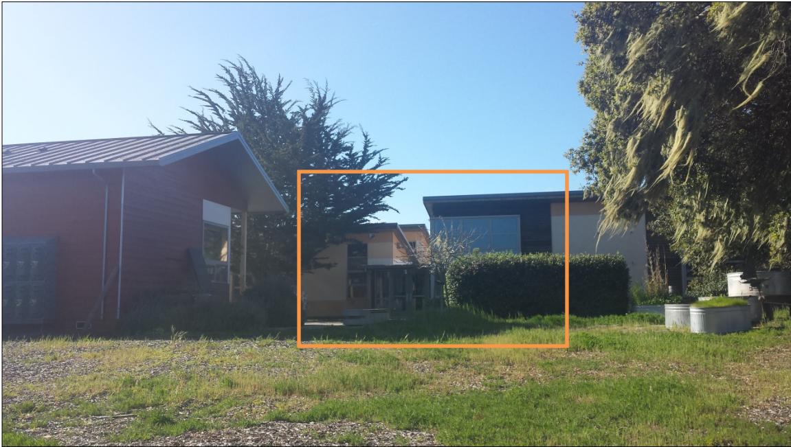
West end of Bldg. 400 (from the north) showing approximate location of sheds
