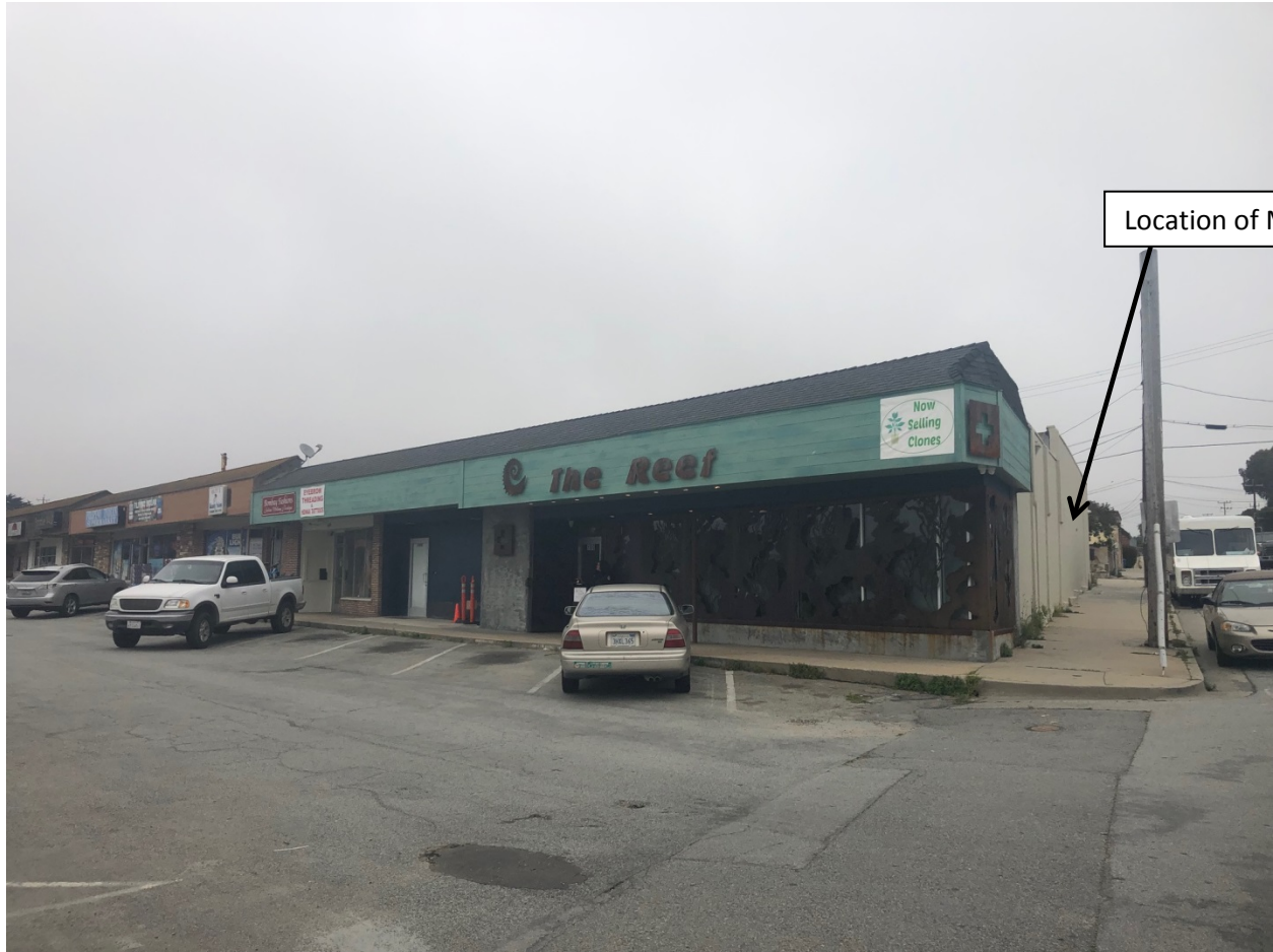
View of front façade of "The Reef" facing Fremont Boulevard
