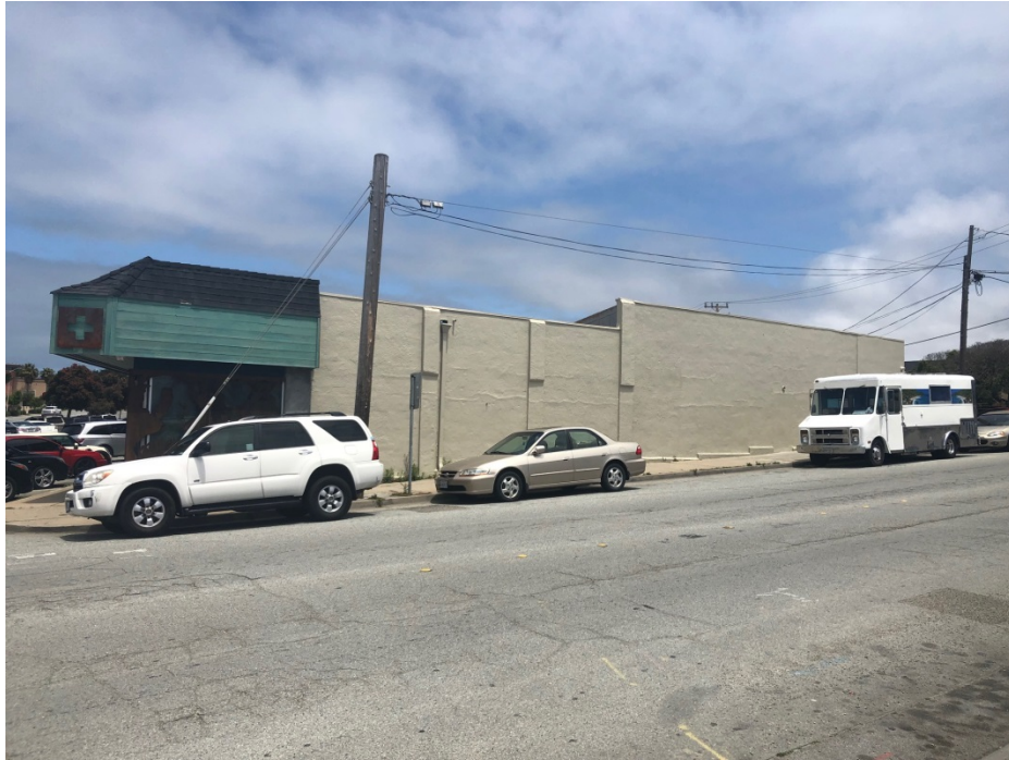
View of wall from La Salle Avenue elevation looking northeast
