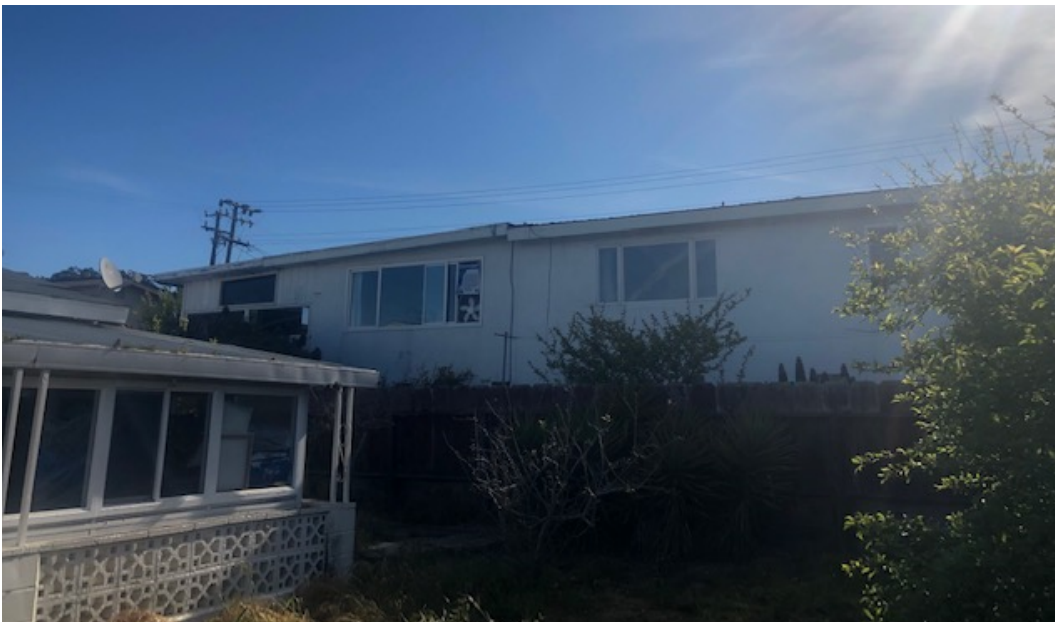
Rear yard windows of 1893 Nadina, as taken from south side yard of 1892 Juarez
