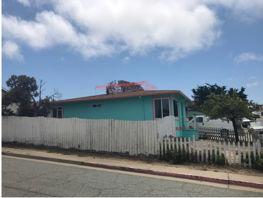
View of dwelling looking south
