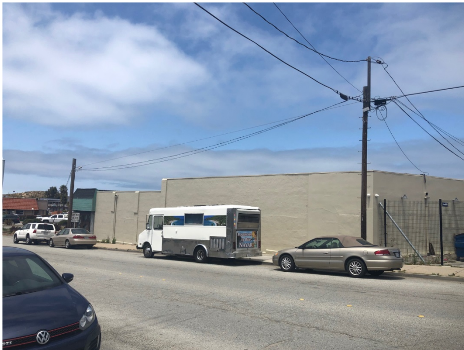
View of wall from La Salle Avenue elevation looking northwest
