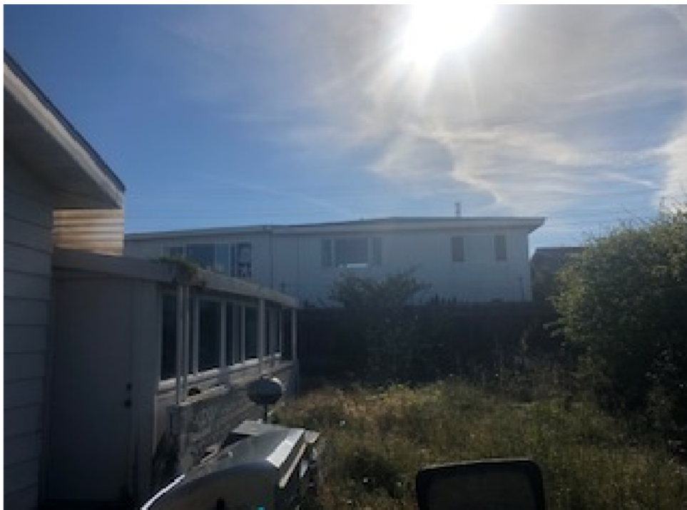
Side yard view of 1892 Juarez, with 1893 Nadina rear windows shown
