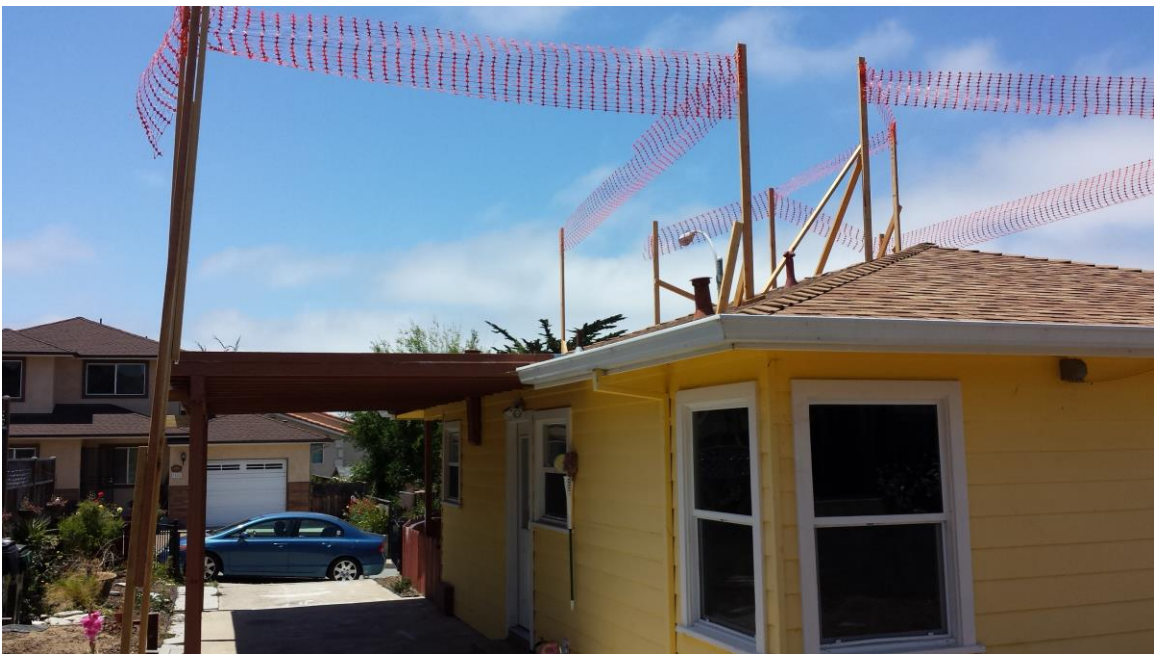
View from rear yard looking towards street through carport
