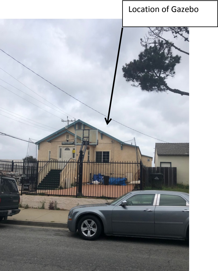
View of front façade from Elm Street
