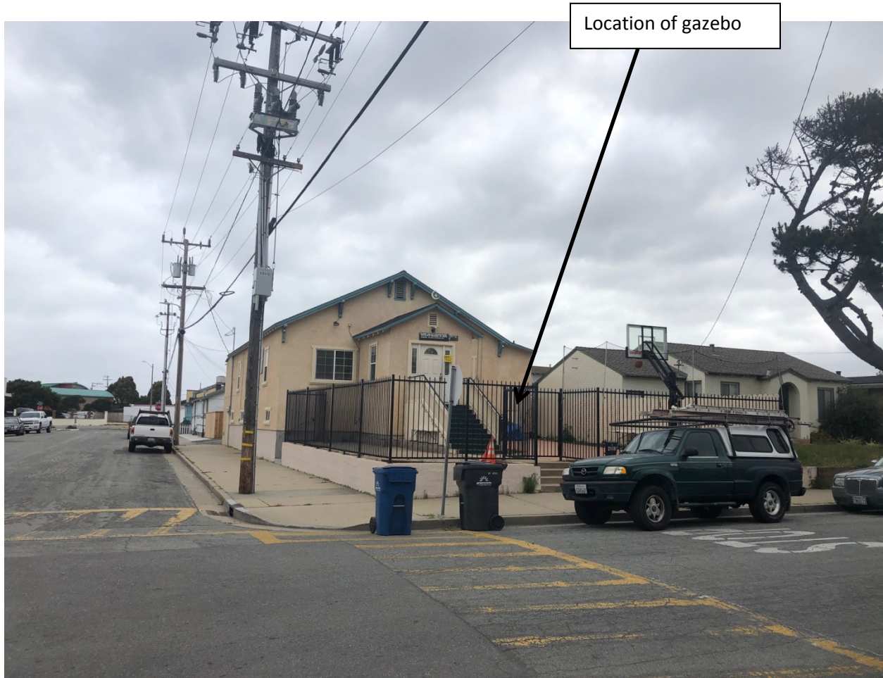
View of front façade from Imperial Avenue and Elm Street
