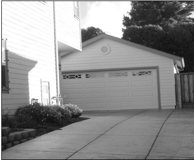
“Detached rear garages and alley-loaded garages are encouraged”
