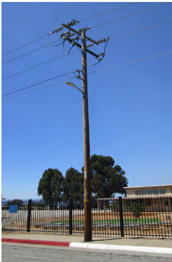
Pole is on Plumas Ave.
