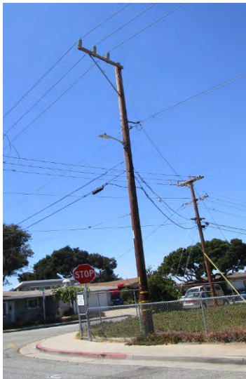
Pole is on intersection of Plumas Ave & Tweed St.
