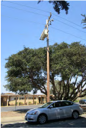
Pole is on Plumas Ave.
