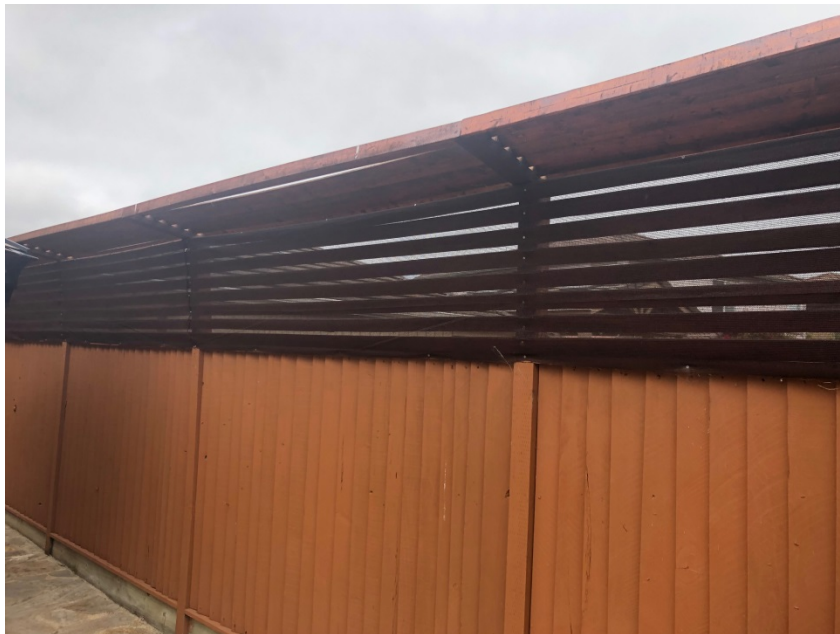
View of fence extension showing curvilinear top section
