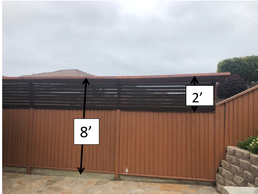
View of fence extension looking west toward 4825 Peninsula Point Drive
