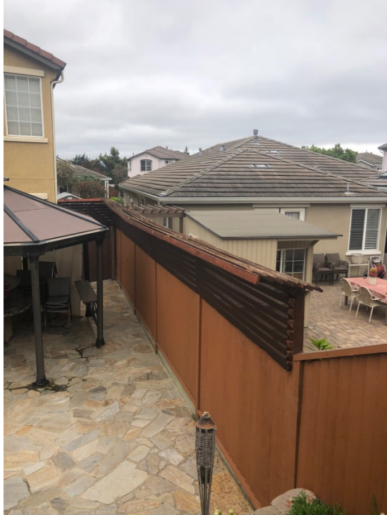
View of fence extension at grade on rear yard
