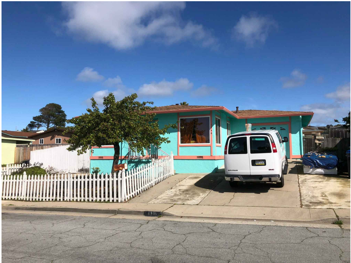
STREET VIEW OF HOUSE & GARAGE LOOKING EAST
