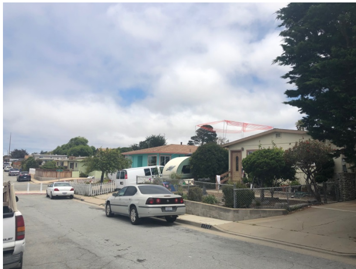
View of dwelling looking north
