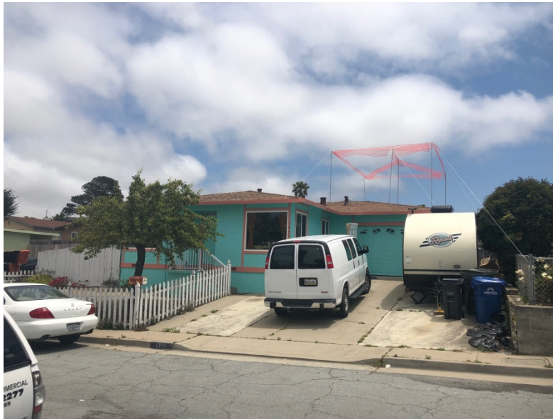
View of front facade
