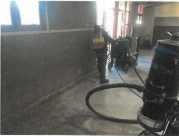
Community Room start to finish from vinyl to custom colored stained concrete.
