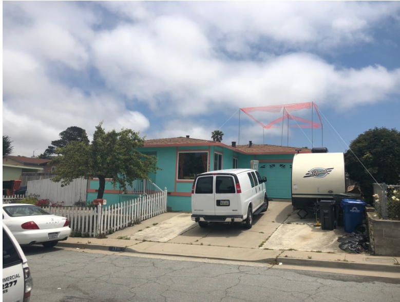
View of front facade
