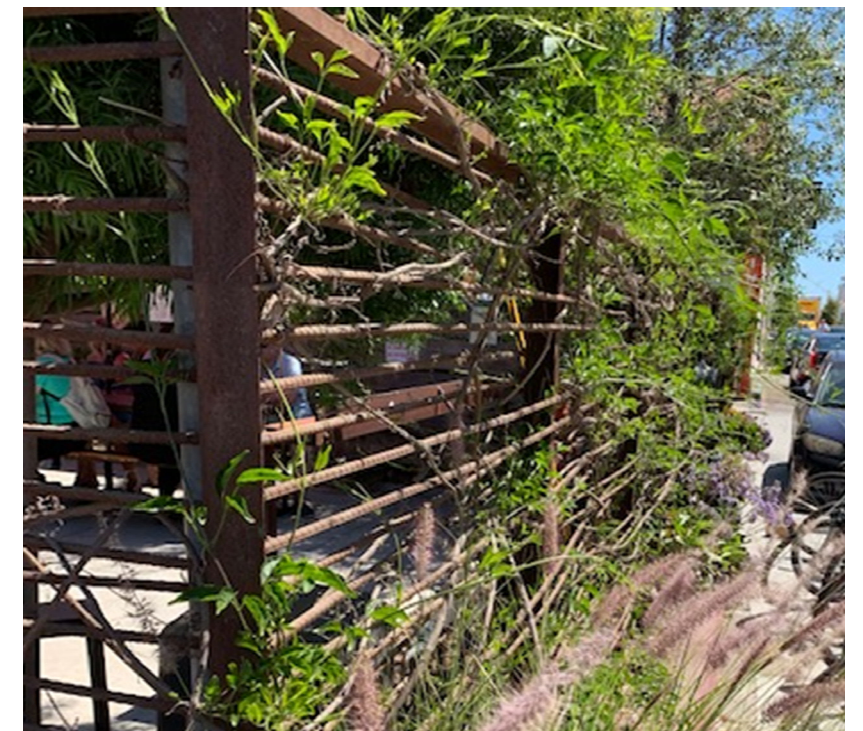
PERMIMETER FENCE. REBAR AND STEEL
