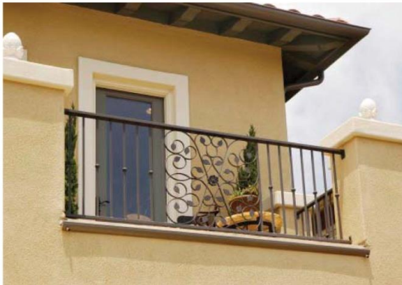
Wrought iron railings
