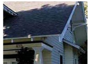
Flat tile roof
