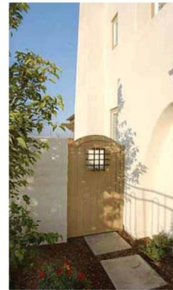
Gates with wrought iron elements
