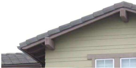
Exposed rafter tails
