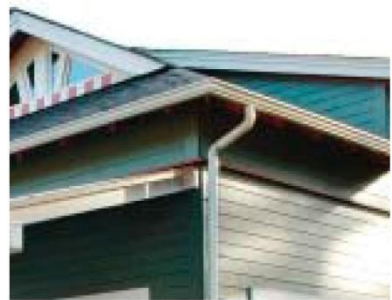
Wide projecting roof forms
