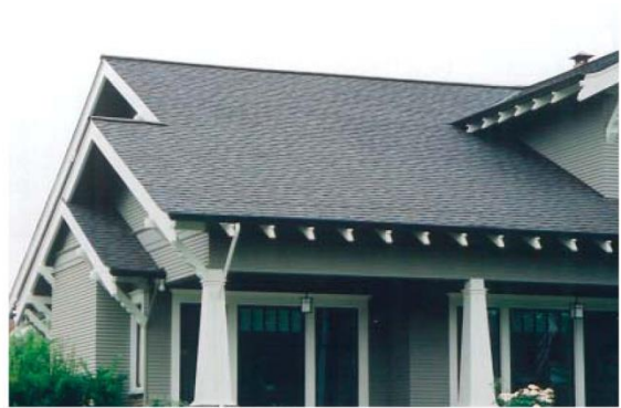
Exposed rafter tails
