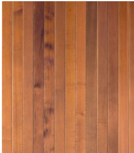
CEDAR SIDING INSTALLED VERTICALLY ON INTERIOR OF ENTRANCE
