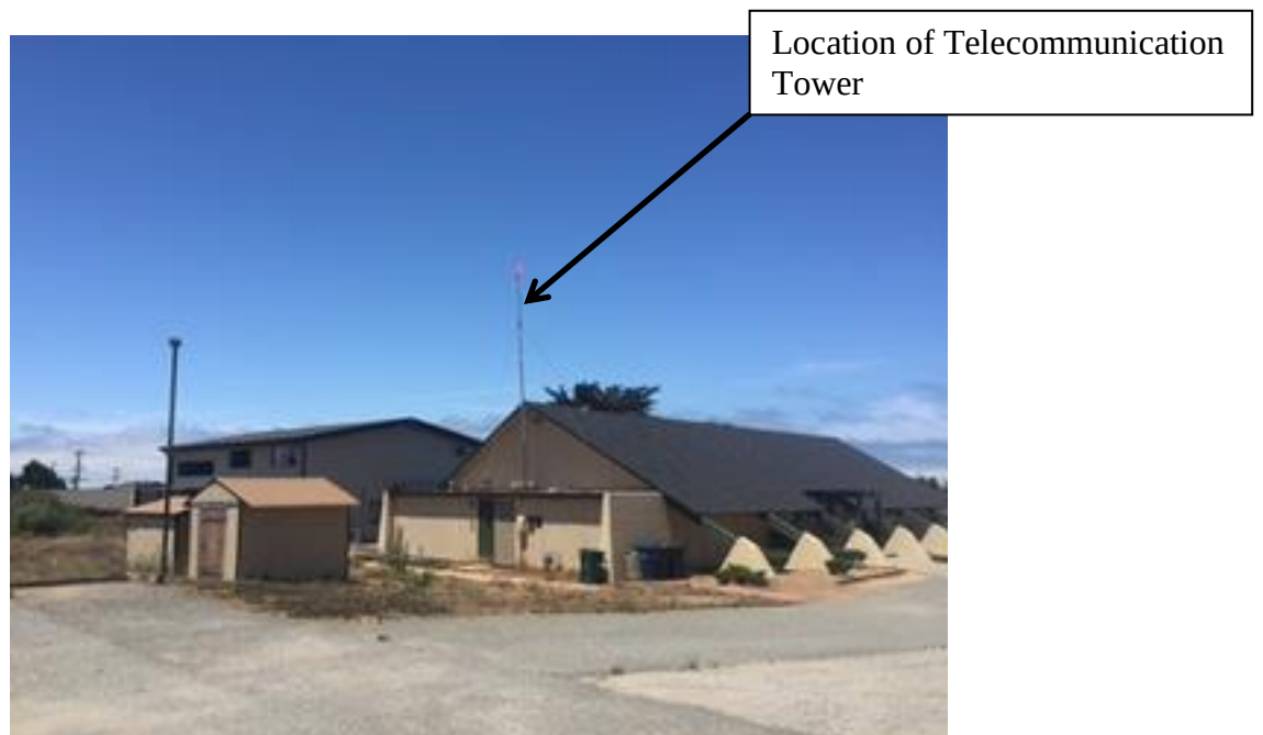
View from the rear parking lot on east side
