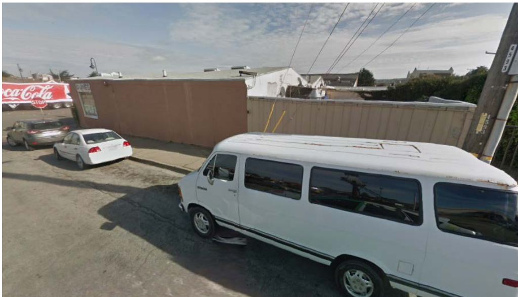
View of Side façade on Contra Costa Street
