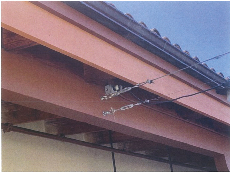
Example of bolting stain-less steel cable to fascia boards.
