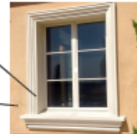
Stucco Trim and Sill
