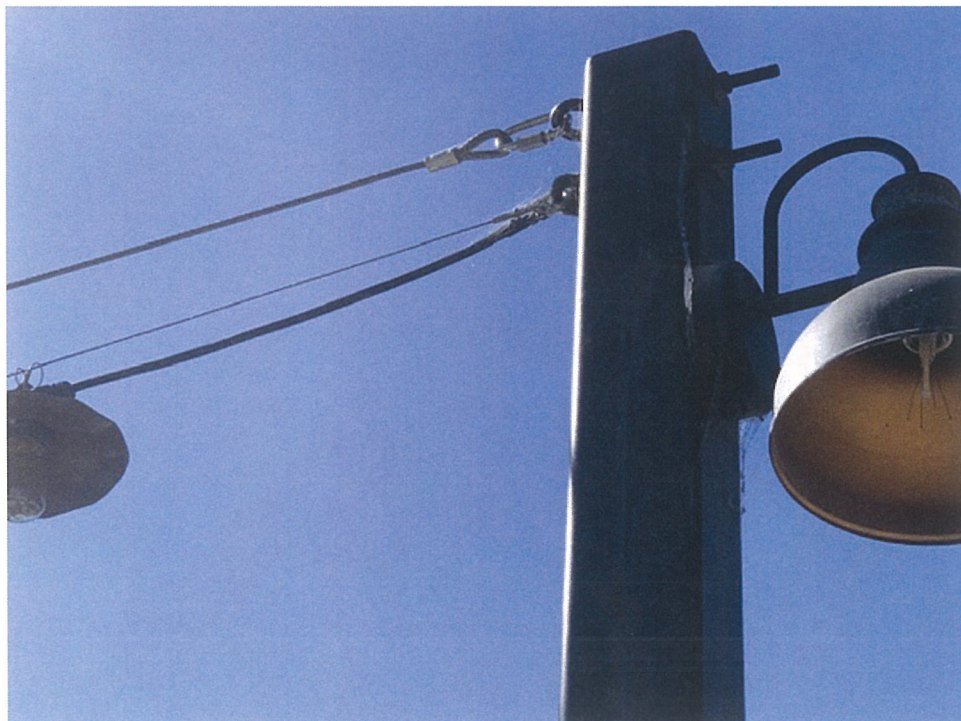
Example of 4 x 4 post with anchor of stain-less steel cable & led light strand.
