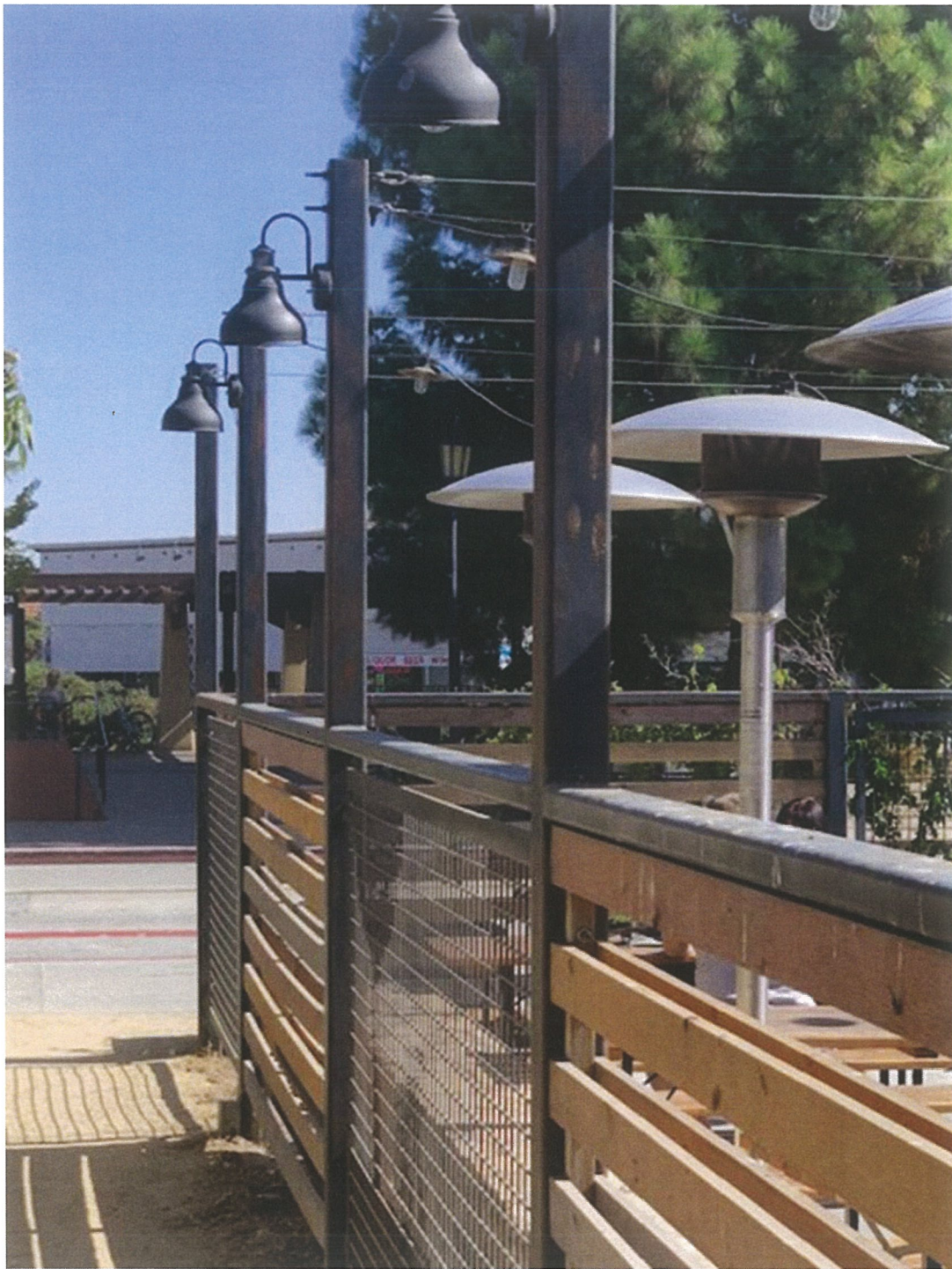
Example of 4 x 4 post with anchor of stain-less steel cable & led light strand.
