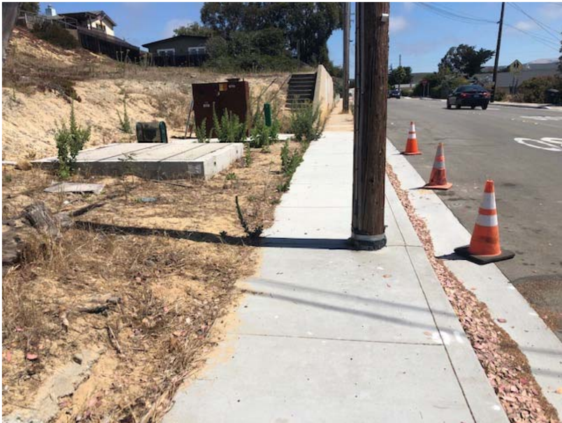
2019 – CalAm’s vault at location of requested red curb East of Luzern.
