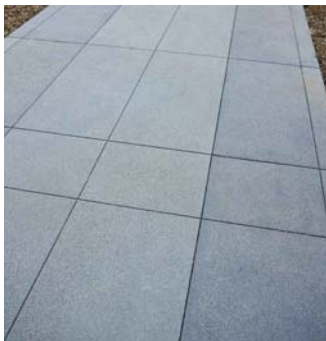
SAWCUT GREY CONCRETE AT PEDESTRIAN WALKWAYS
