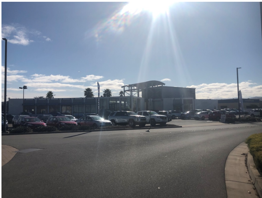
View from northwest corner looking south
