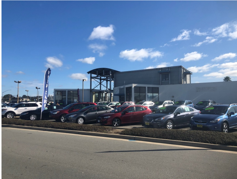
View from southwest corner looking north
