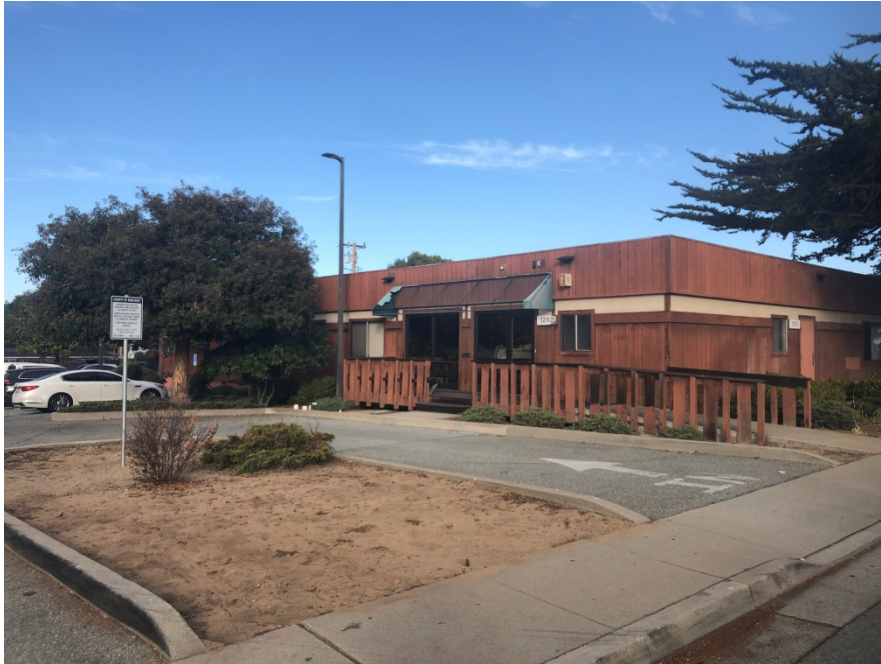
View of front façade facing parking lot
