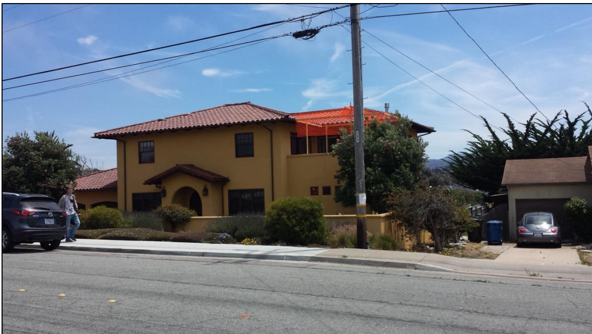
Street view of open deck that will be enclosed
