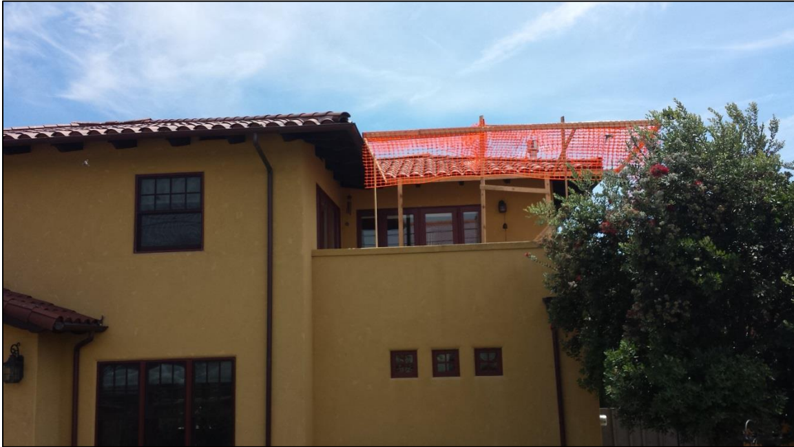
Close up of open deck that will be enclosed
