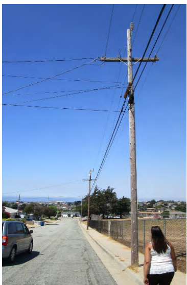
Pole is on Tweed St.
