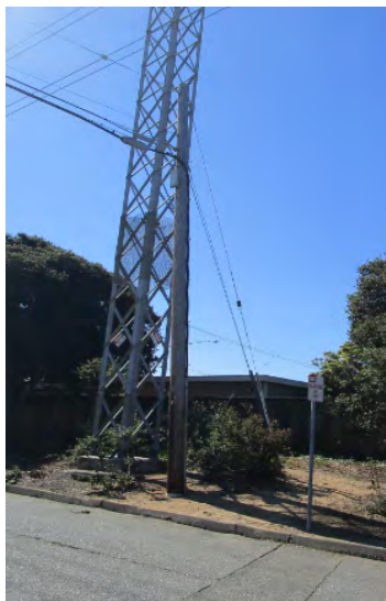
Pole on Intersection of Plumas Ave & Noche Buena St.
