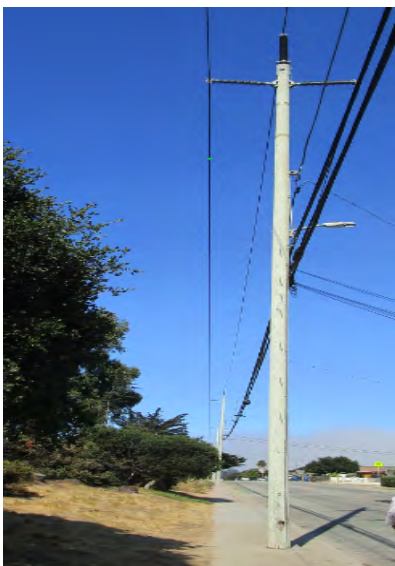
4th pole on Kimball Ave.
