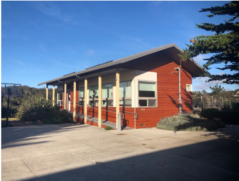
View of Existing Modular Building
