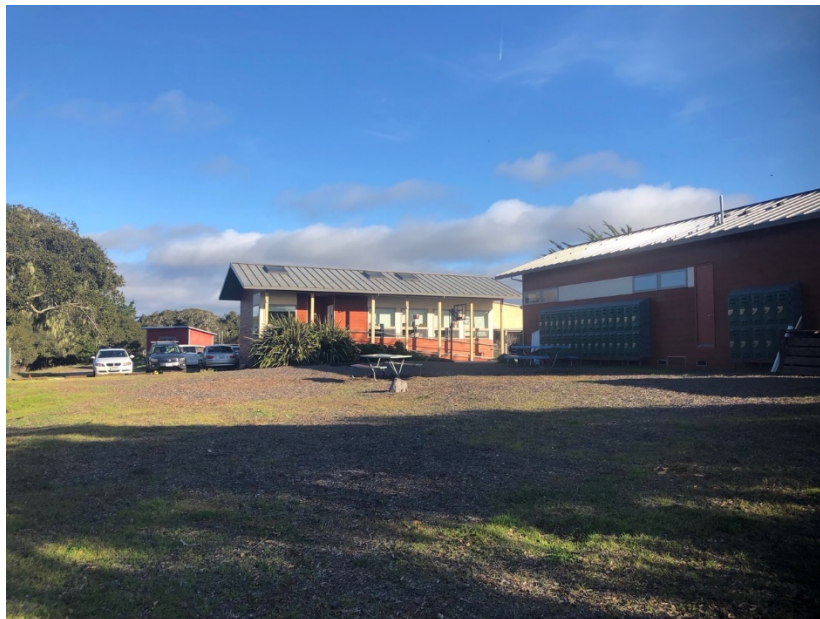
View of Location for proposed Modular Building
