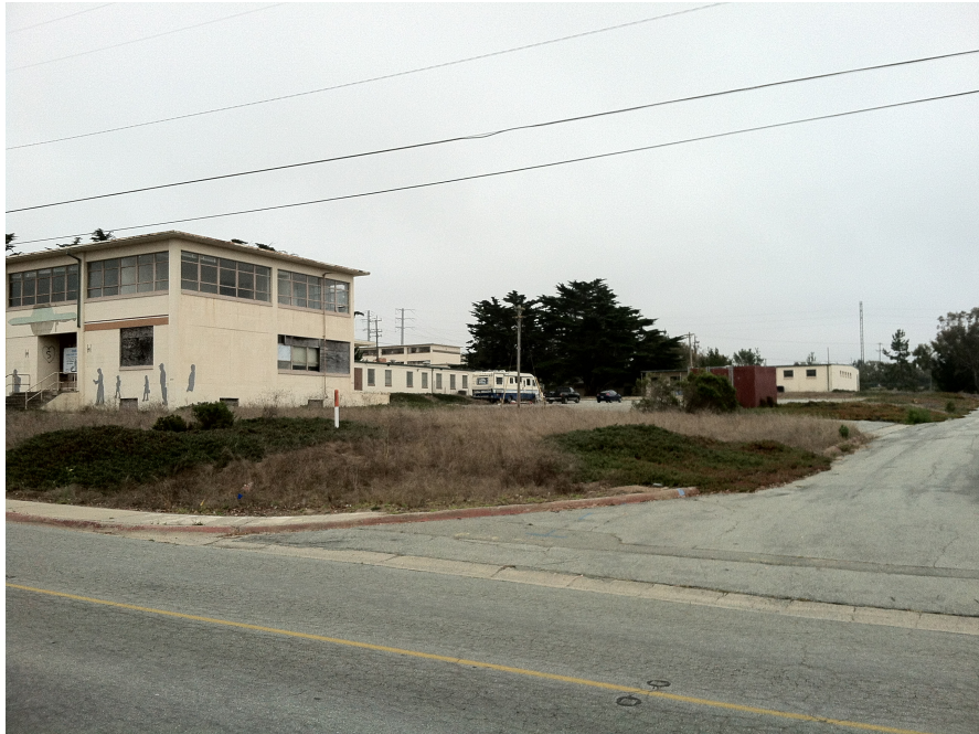
View from northwest corner of the site
