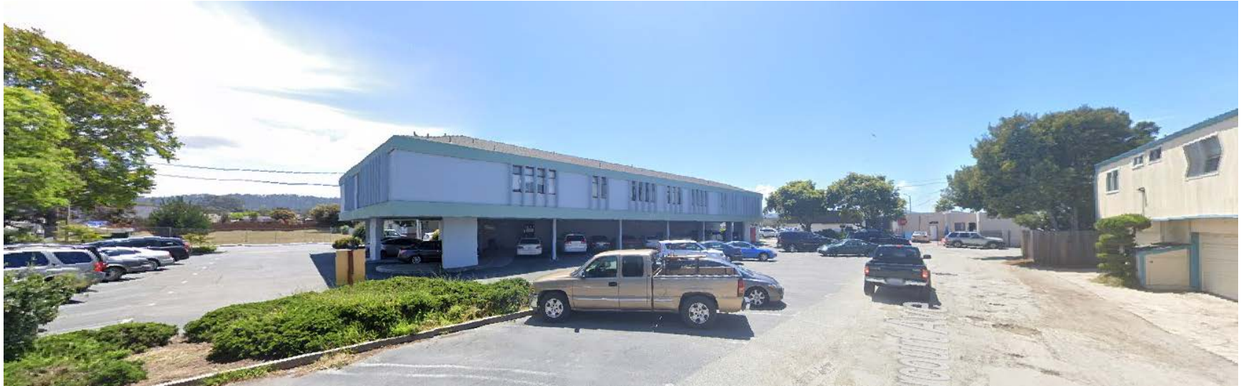
View showing the commercial building, parking lot, and Harcourt Avenue right-of-way, as well as the multi-family use to the north.
